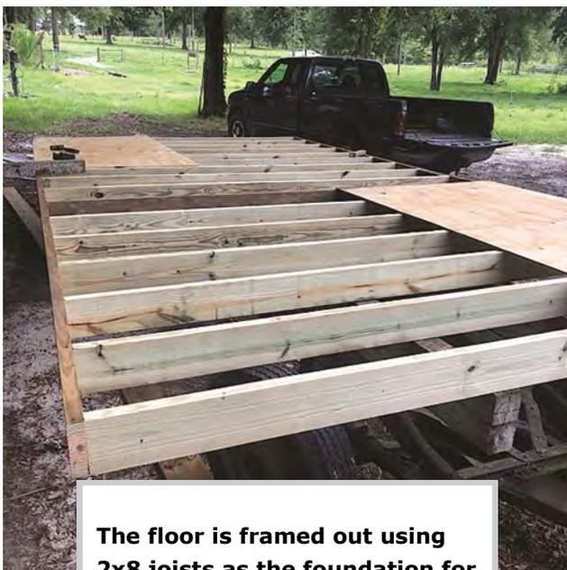
**The floor is framed out using 2x8 joists as the foundation for the mobile brooder.**
